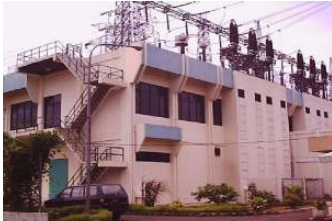
Gambar 15.10. Gedung Kontrol (Control Building)
