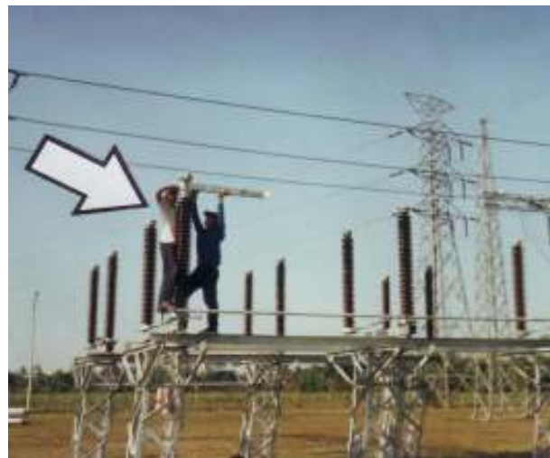
Gambar 15.6. Disconnecting Switch
