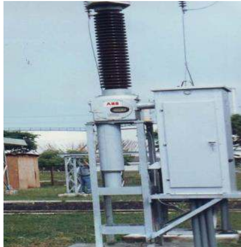
Gambar 15.5. Circuit Breaker
