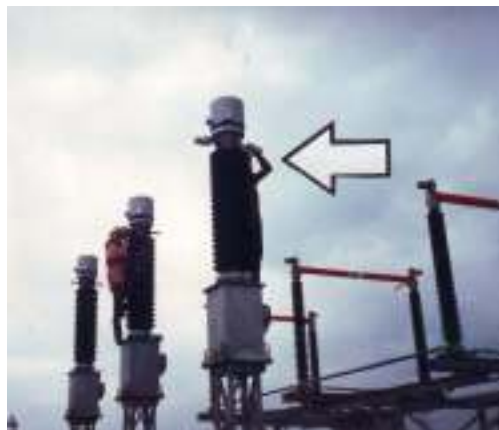
Gambar 15.8. Current Transformer (Ct)
