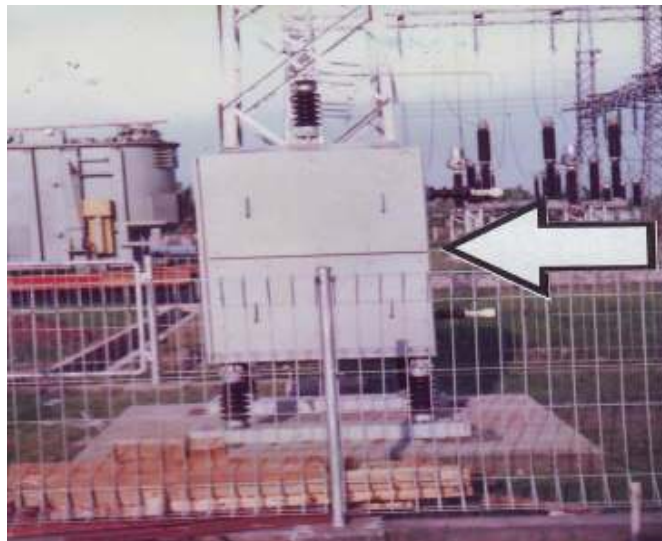
Gambar 15.1. Neutral Grounding Resistance (NGR)
