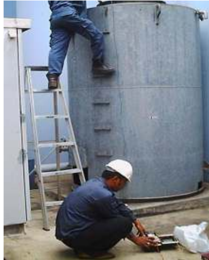
Gambar 15.2. Neutral Grounding Resistance (Liquid)
