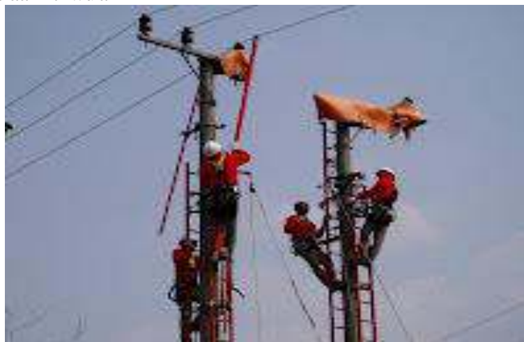
Gambar 14.31. PDKB Metode Rubber Gloves
