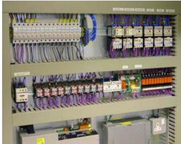
Gambar 2.20. Sub Distribusi Panel
